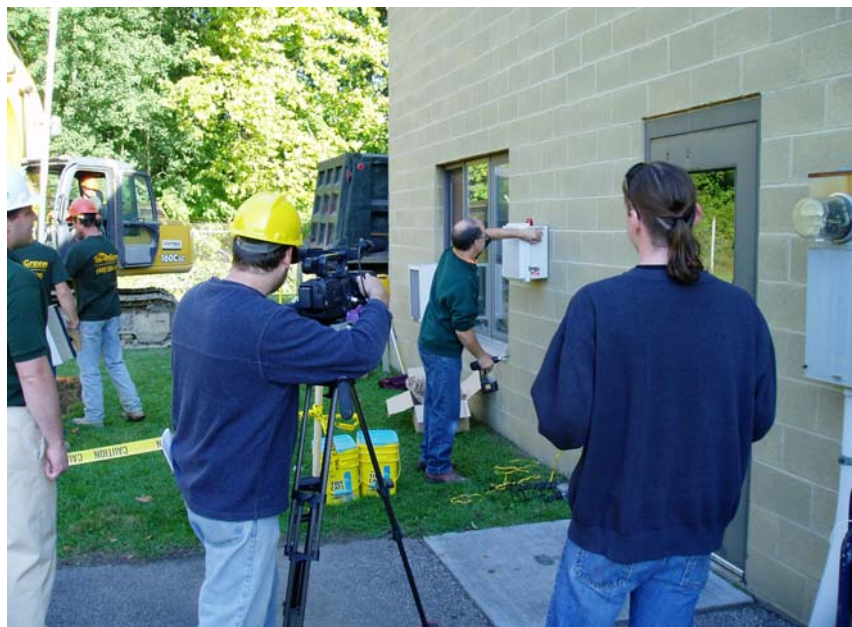
Filming electrical work
