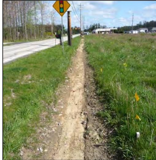
**Figure 3 and Figure 4.** Established vegetation on the fore slope, back slope and roadside berm (left, Figure 3) using wood fiber hydro mulch at the Bass Lake Road demonstration site in Munson Township, Geauga County. Failed vegetation with paper hydro mulch application at Bass Lake Road (right, Figure 4).
