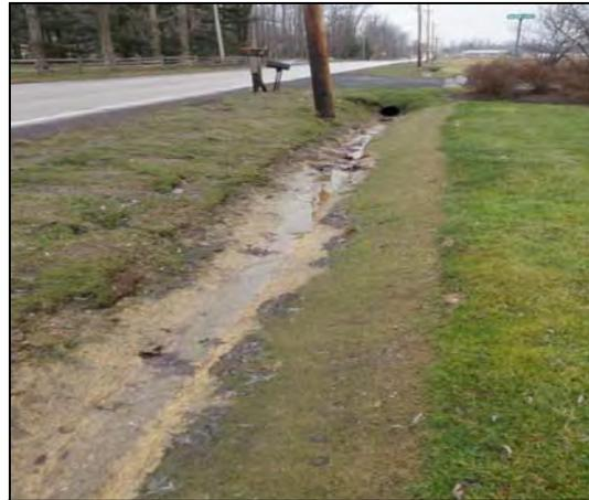
**Figure 6.** Bass Lake Road, Northern Treatment Zone January 2012 germination. Note hydro mulch coverage of soil surface.
