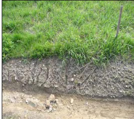
**Figure 8.** Bass Lake Road, Northern Treatment Zone close up photo of back slope showing rill erosion and rock pedestals.
