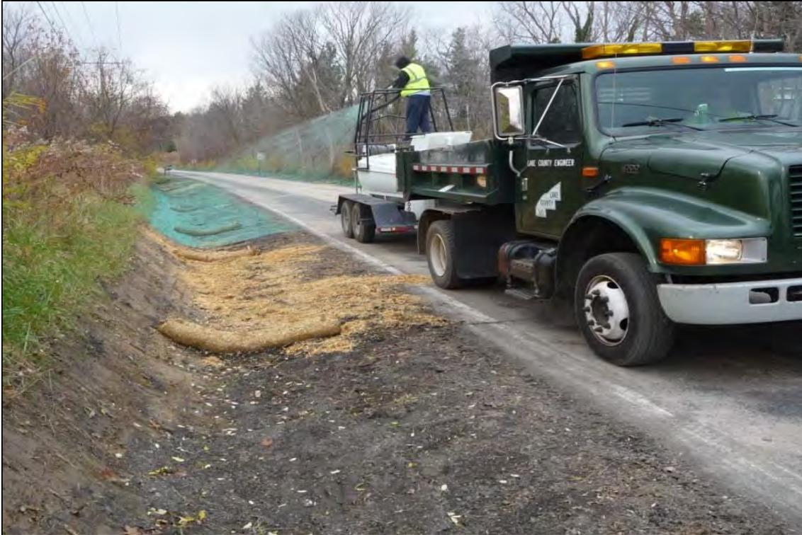
**Figure 2.** Lake County Engineer application of straw wattle and wood fiber hydro mulch at the Ledge Road demonstration site in Madison Township, Lake County.
