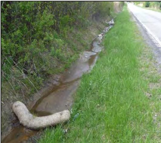
**Figure 15.** Straw wattle trapping sediment. Drainage is flowing from top to bottom in picture.
