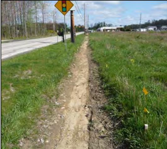
**Figure 7.** Bass Lake Road, Northern Treatment Zone April 27, 2012 showing failed germination on fore and back slope.
