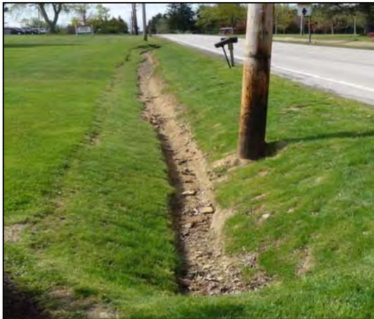
**Figure 5.** Bass Lake Road, Northern Treatment Zone April 27, 2012 full germination of fore slope, back slope and berm.
