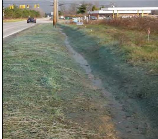
**Figure 4.** Bass Lake Road, Northern Treatment Zone receiving BMP installation on November 17, 2011.
